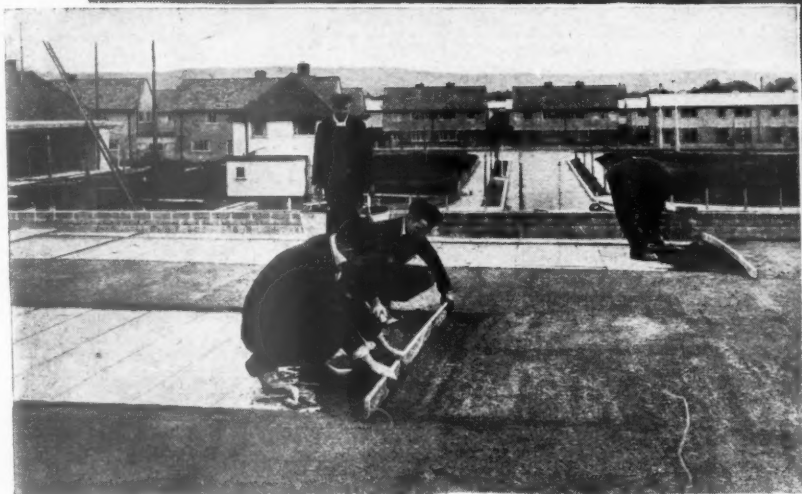
KISOL Vermiculite ready mixed screed being applied to the roof of Gabalfa School, Cardiff.
