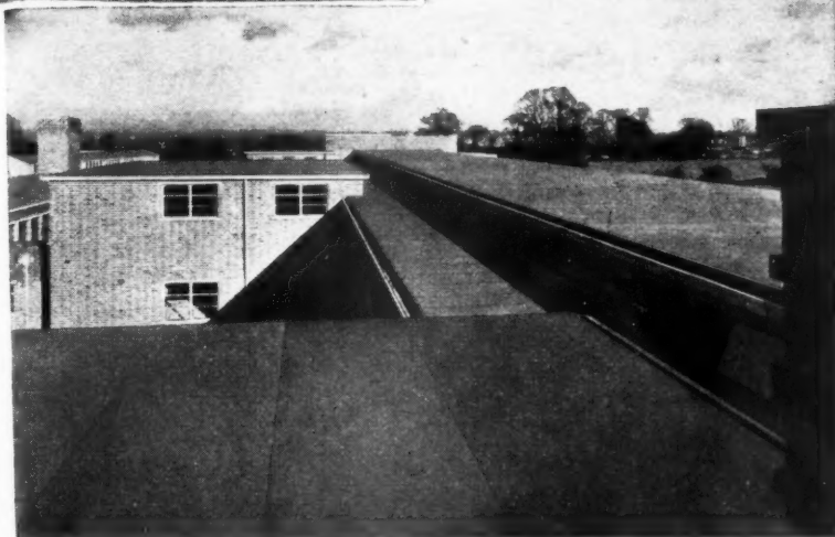
Roof of Hanbridge School, Chester, screeded and completed with KISOL Vermiculite.
