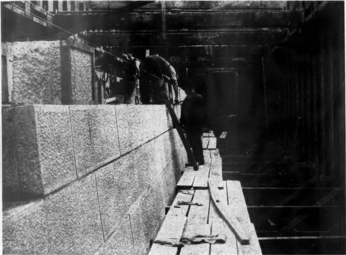
De Lank Granite being used in the construction of the South Bank river wall.
