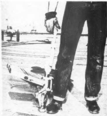
Left, a workman guiding with his foot an American automatic nailing machine. Below, spraying liquid vinyl plastic as a roof covering. Right, the General Electric Co. of New Jersey's combined heat pump and air-conditioning plant.
