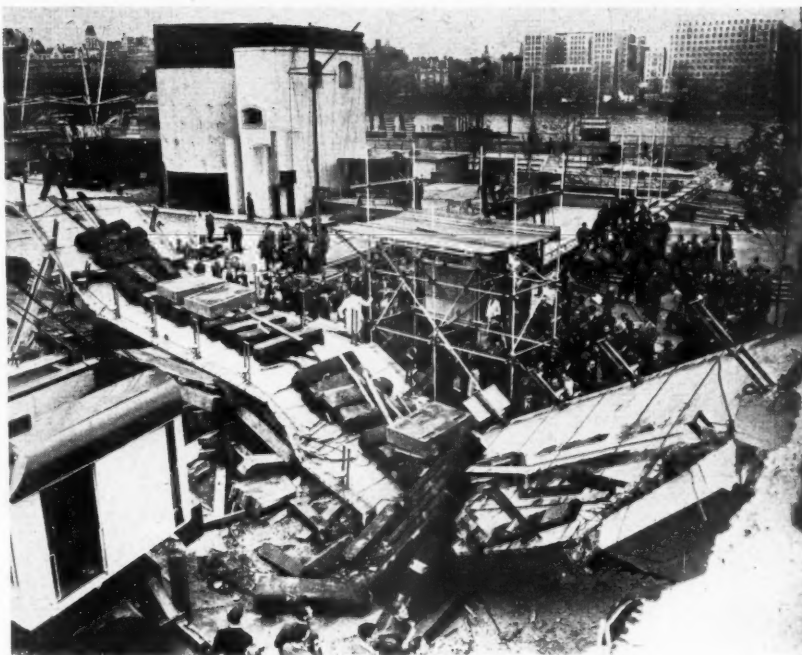
The prestressed concrete footbridge on the South Bank collapsed last week during over-loading tests, after 88 tons had been placed on it. See ASTRAGAL's note on this page.
