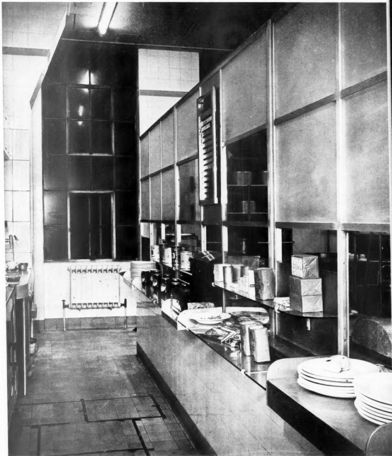
The upper part of the screen is of glass framed in aluminium: there are movable aluminium shelves on the kitchen side and fixed glass shelves between the hatches on the serving side of the screen.
