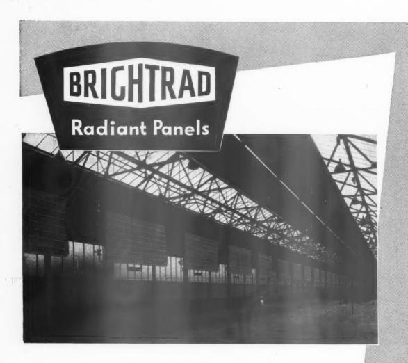
Controlled, comfortable working conditions are assured in industrial buildings by BRIGHTRAD Radiant Panels. Designed for surface temperatures of 200° — 250°F, these panels give a pleasant working environment. They make for economy in maintenance and running costs.
