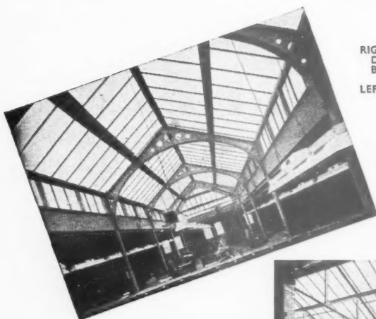
BELOW: Roof Glazing over Joiners Shop of Messrs. Harland Wolff Ltd. North Woolwich.
