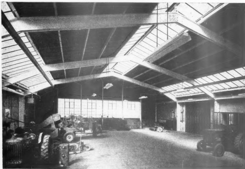
Left, the repair shop, which is spanned by a welded arched rib steel frame. Below, the entrance hall; the showroom on the left behind a glass screen.
