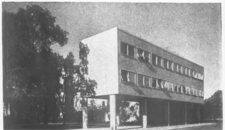
Top, looking north from the loggia under the office block towards the transformer cell. Right, looking north-east at the raised office block.
