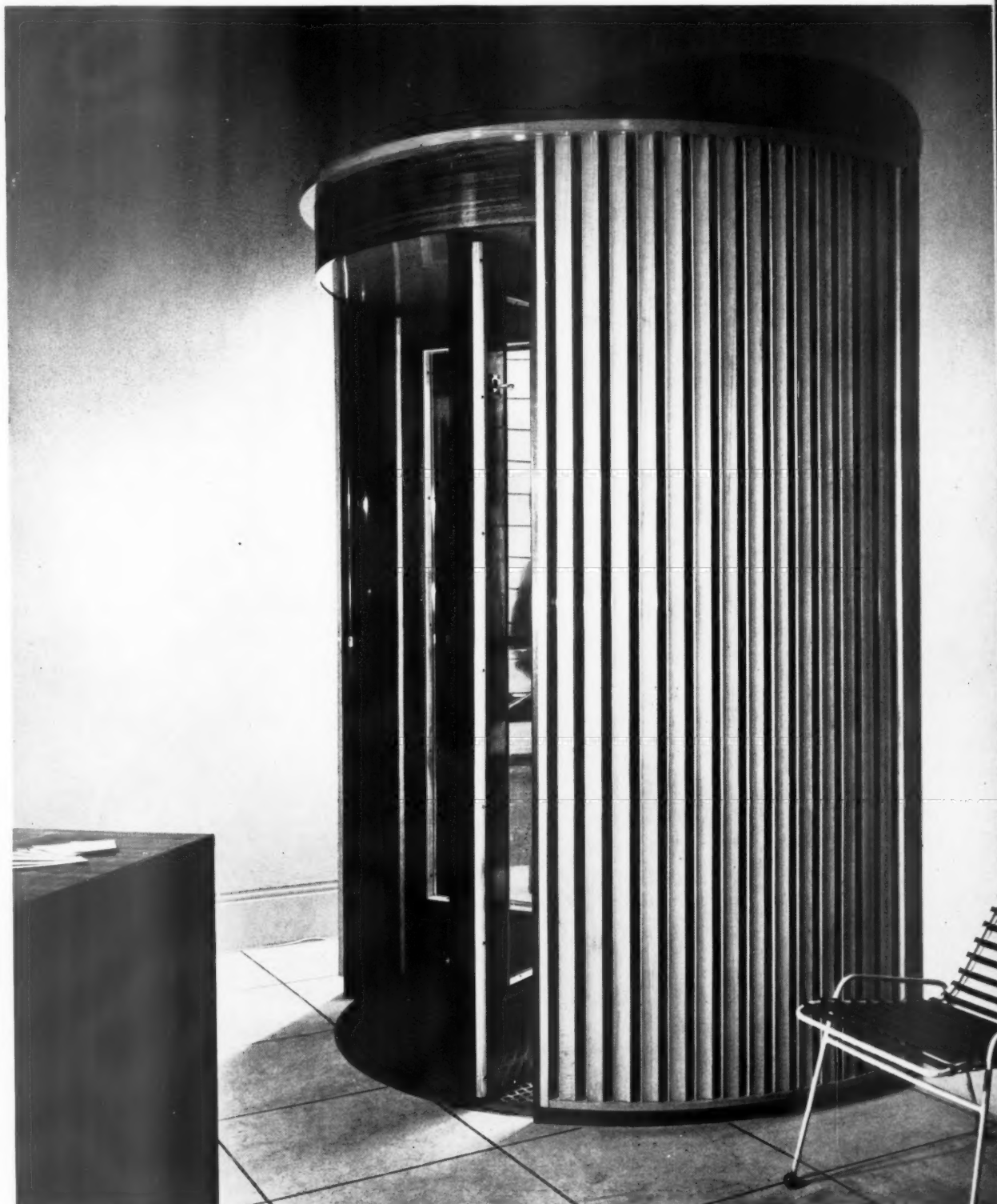
The doors are in natural mahogany and the side casing is panelled on the outside in vertical moulded strips of obechi.
