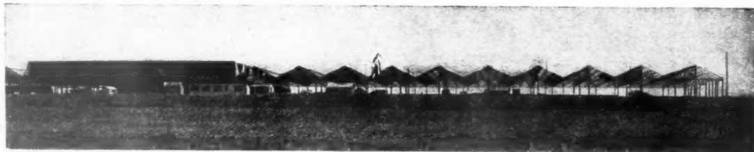
Portion of Works for Messrs. de Havilland Propellers Ltd., Lostock
