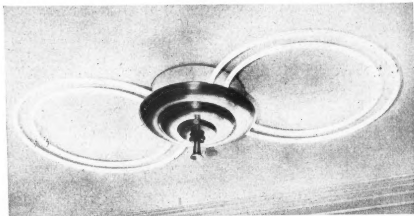
Fig. 5, specially designed G.E.C. fitting, supplied to order, for Osram cold cathode tubes totalling 30 ft. in length. All the gear is contained in the drum, which is cellulosed cream. The decorative spinning is satin silver, with a gilt finial. Consumption is 250 W.
