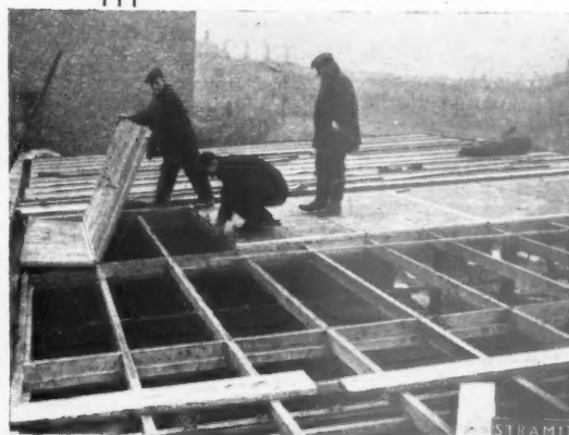
Illustrations show two typical examples of Stramit in use as a partitioning and roof decking.
