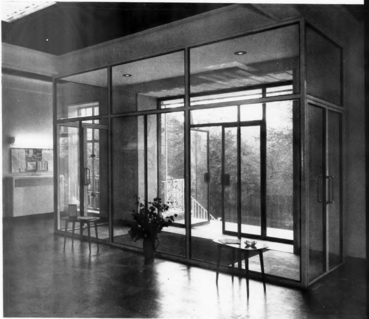
The entrance doors are framed in bronze and the screen in painted steel, with all glazing beads in hardwood.
