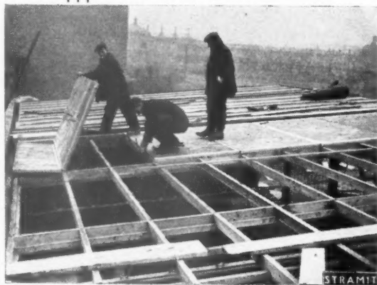
Illustrations show two typical examples of Stramit in use as a partitioning and roof decking.
