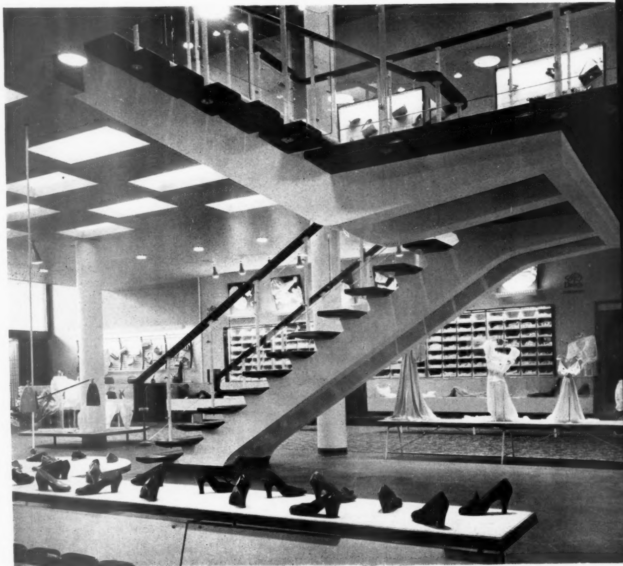
The staircase is supported on two reinforced concrete carriage beams and the hardwood landing is treated in the same way as the treads, having a wide overhang through which the balustrade standards are bolted.
