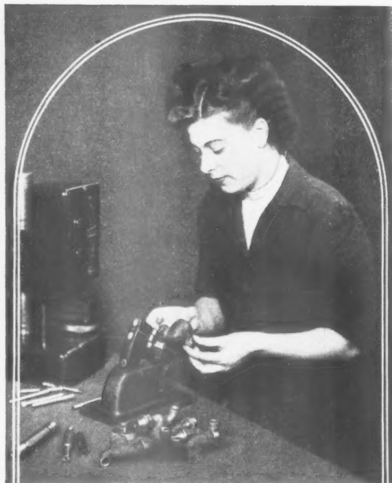
Screw and spindle gauging
