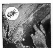
A rafter in the roof of Chichester Cathedral showing damage by the Death Watch Beetle.
