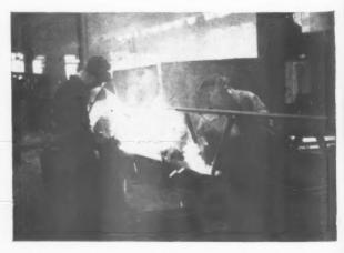
Above, Fig. 1, a steel lattice beam being welded in the works. Left, Fig. 2, a cranked lattice beam (not used at Wokingham) being galvanized by dipping in multen zinc.
