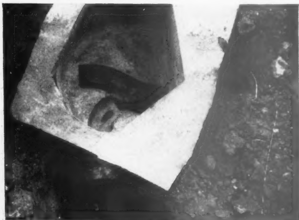
Fig. 16, part of the fibrous plaster ceiling which has recently been developed and which is being fixed in the hall. The pattern derives from the holes which are cast into the panels, behind which an acoustic absorbent is fixed. Each panel rests on a rebated fibrous plaster rail which is wadded to the steelwork.
