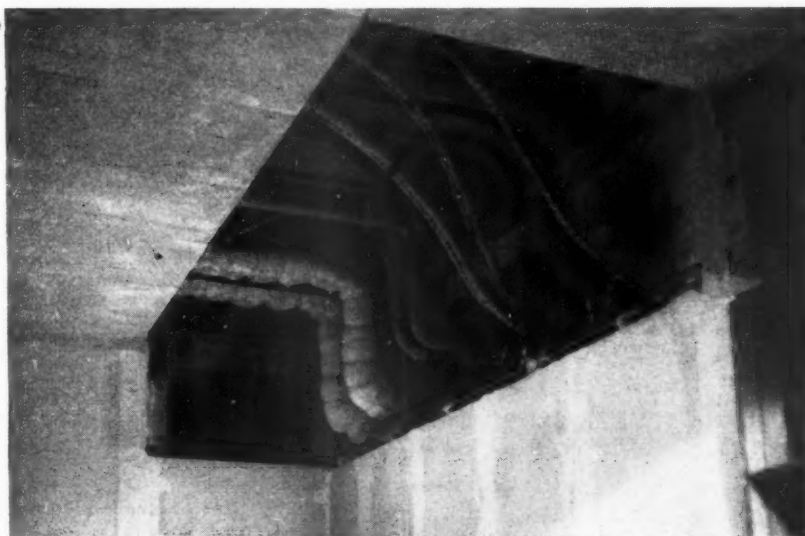
Fig. 8, part of ceiling, showing heating pipes and electric cables in interspace.
