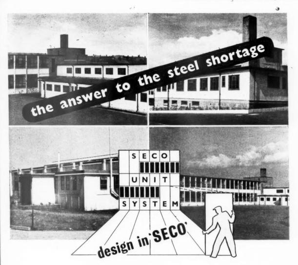
The SECO system of unit construction makes it possible for widely differing types of building programmes to go forward in spite of steel shortage. The need for structural steel is eliminated by the use of SECO AERO stressed skin beams and columns, prefabricated in suitable spans, and immediately available from stock.
