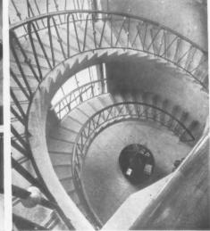
Main staircase of reinforced concrete cantilevered from main frame
