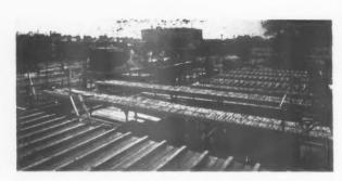
Left, 110-ft. T-section secondary beams used for hangars at London Airport, composed of 7-ft. lengths, prestressed on "string-of-beads" principle. Above, progress photo of school at Paragon Road, Hackney (Howard V. Lobb and Partners; engineers, Samuely in conjunction with Messrs. Bullen & Partners), showing floor system using prestressed soffils, inverted T-shaped precast units of or dinary concrete, wood-wool and 12-in. screed.
