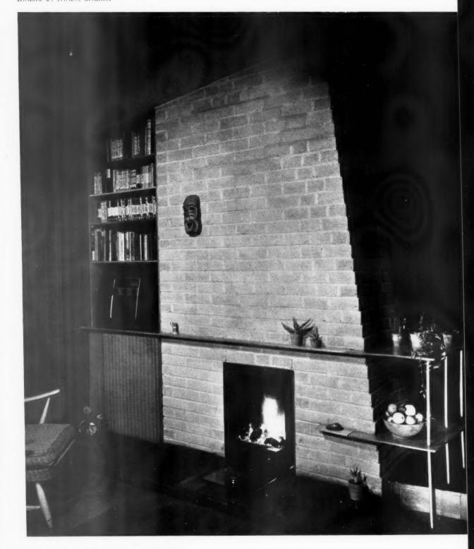
The fireplace in the living room is provided with air from ducts under the floor and heats the dining recess by means of a warm air outlet at the back
