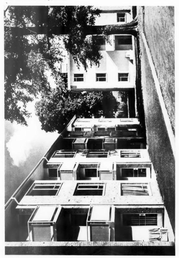
The balconies are paved with concrete tiles and the hainstrading is formed from fluted asbestos-cement pusels with handrail and corner posts of steal tube
