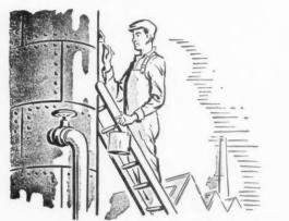
The paint trade is using our METALLIC LEAD PIGMENT for this kind of job. In a few words, Spelthorne Metallic Lead Pigment is 99.5% finely divided metallic lead in linseed oil or other media. It protects metals from corrosion and wood from decay. It flows easily, covers well and forms the base of chlorinated rubber paints. Lead is now free of control, and supplies are easier. Protection of property with Metallic Lead Paint will save maintenance costs. Samples and prices from:-
