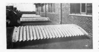
The use of plastics in building in 1952. Left, curved corrugated "Perspex" used for rooflights. Below, the primary school at Boreham Wood, Herts. (architect, C. H. Aslin), where glass-fibrefilled hollow plastic panels were used for external cladding, as well as internal partitions.
