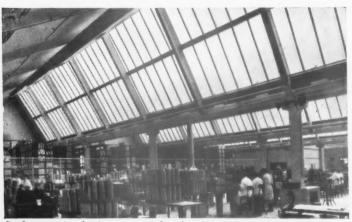
Roof construction showing precast reinforced concrete trusses, purlins and main beams
