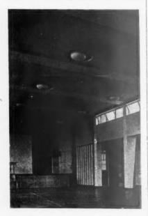
Assembly hall of primary school at Poplar (designed by C. C. Handisyde, in association with Hammett and Norton; consulting engineer, F. J. Samuely). The roof consists of prestressed concrete "soffits" (seen projecting below the suspended ceiling) with trough units spanning between them and a topping of in situ concrete.
