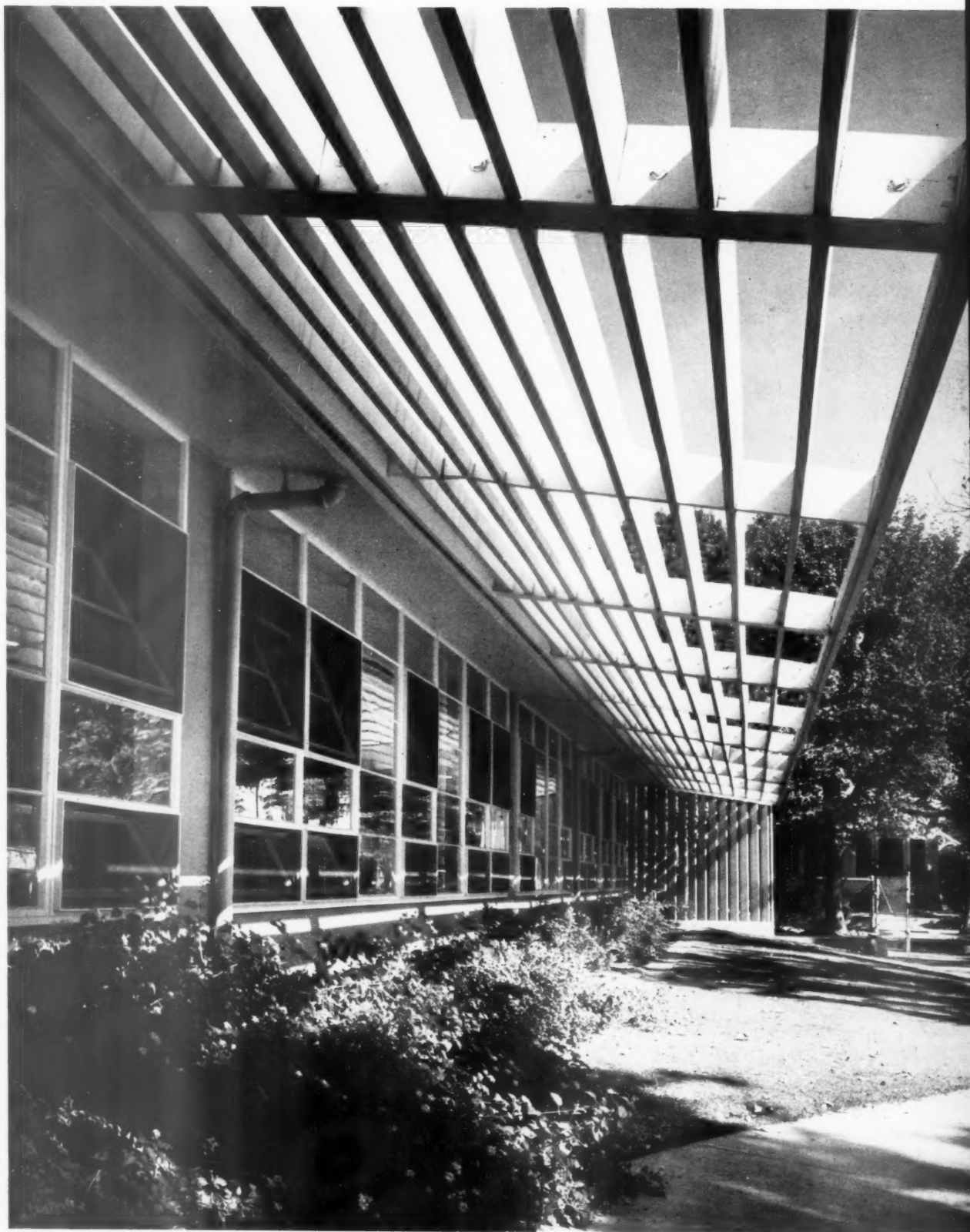
The ends of the steel roof beams, cased in timber, extend to form supports for the redwood louvers.
