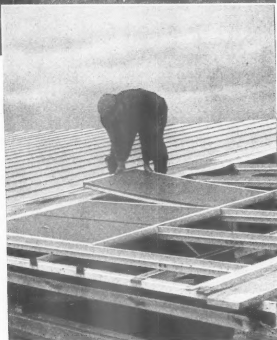
Inset photograph shows Stramit boards and copper cladding.
