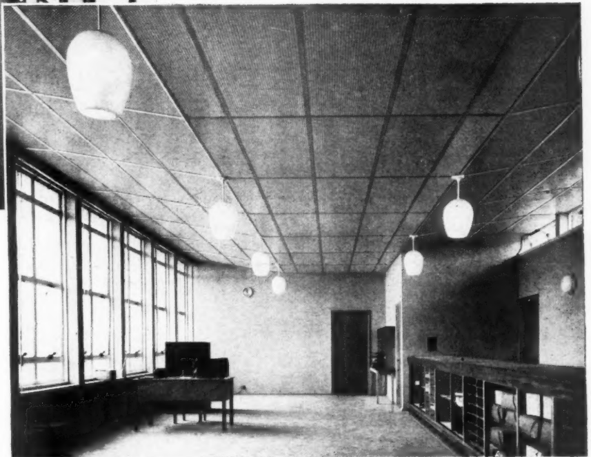
Ceiling lining in TenTest "Rabbit Warren" Acoustic Board fixed by means of our Spring Clip Fixing in Aluminium Section
