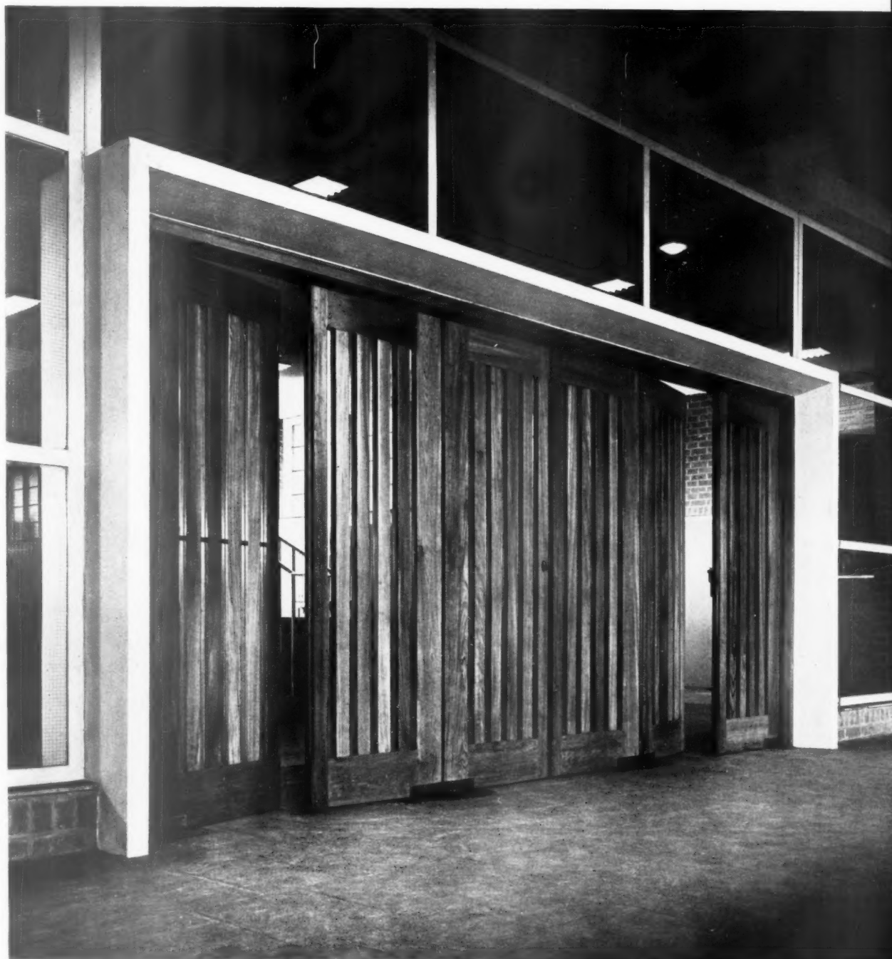
There is no framing between the pairs of doors, which are in teak with narrow vertical strips of glazing.
