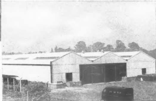
Supplied, erected and sheeted complete on your prepared foundations
