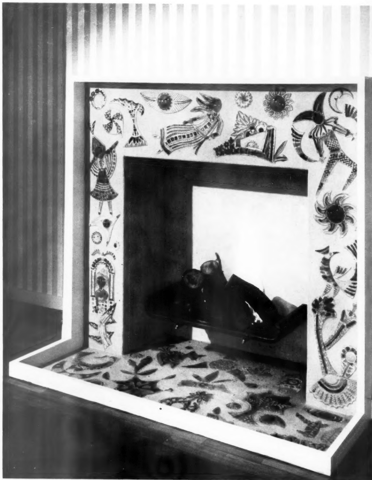
The tile shapes, designed and made by Steven Sykes, are set in rough-textured rendering.
