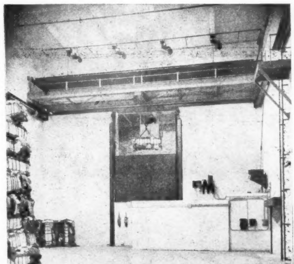
Electrically-operated door and flap for cranes and overhead rail. Above, closed; below, open and in use.
