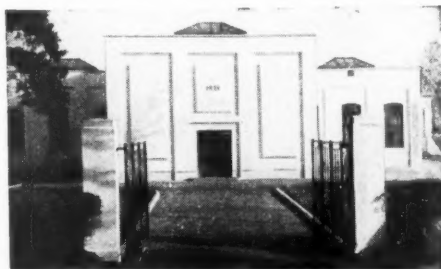
View of a pumping station in Hertfordshire, where Tretolin was used on the Engine House, Workshop and several other ancillary buildings
