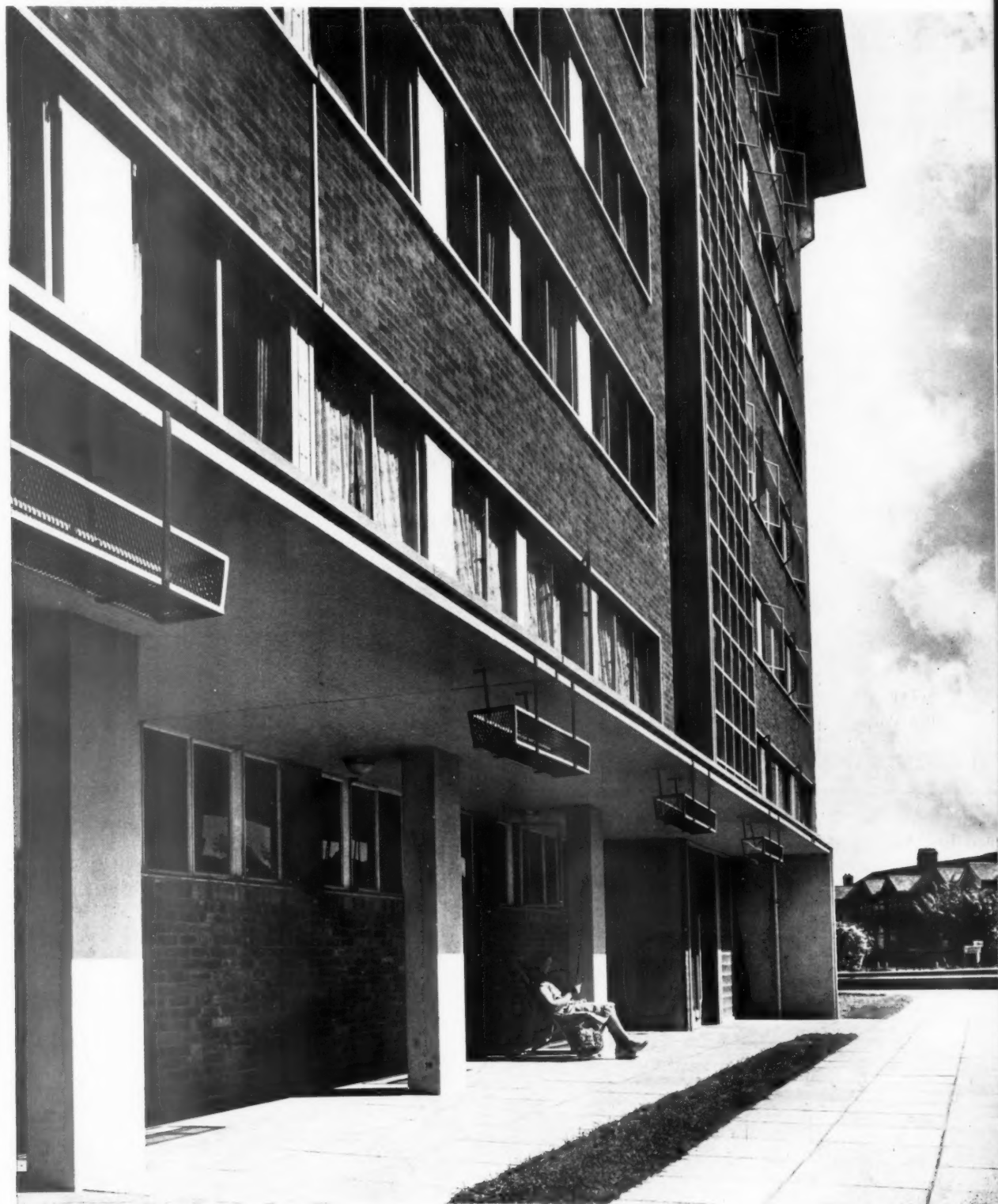
The expansion joint is clearly visible in the brickwork between the windows and continues through the mullion
