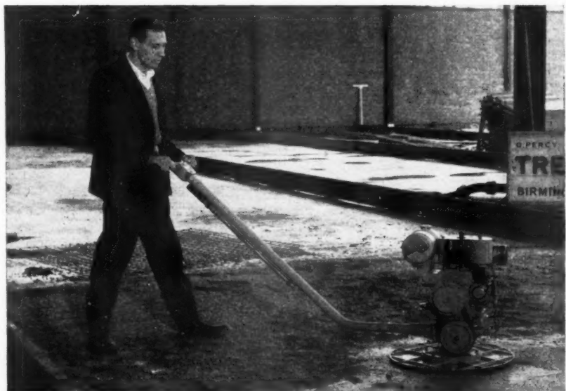
Floor made of no-slump concrete being screeded with mechanical float (petrol-driven model). No great physical effort is required of the operative, and the finish is good enough to receive flooring direct.
