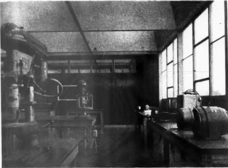
Left, the electrical workshop. Top lighting is from monitor roof lights, under which is an "egg-crate" ceiling on a 10-ft. grid, with fins 5 ft. deep. Below, corridor on the first floor of the two-storey block. This corridor is carried on steel brackets cantilevered from the main steel frame.
