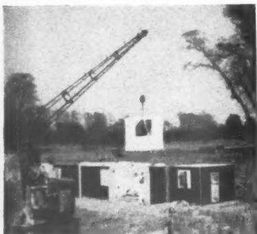
Above, one of the precast gypsum-plaster panels being lowered into position. Below, R. Fitzmaurice, consulting civil engineer to the War Department and the technical editor of the JOURNAL (facing camera) and C. C. Handisyde, consulting architect, discussing the experiment with representatives of the War Department.
