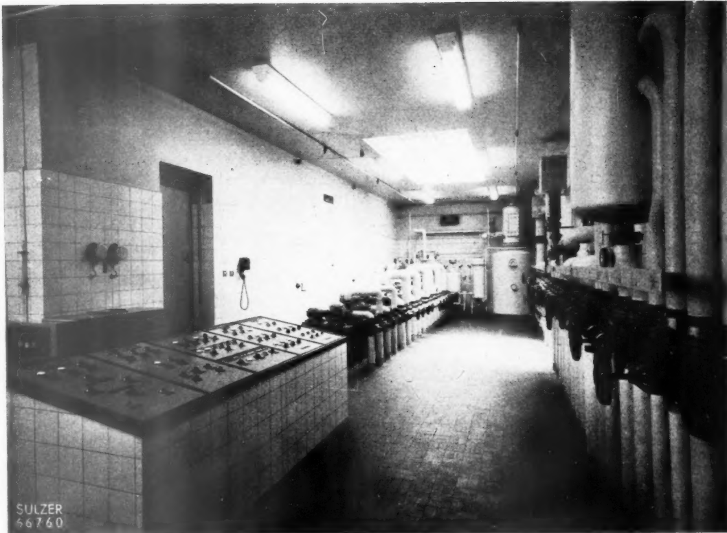
Switchgear and regulating equipment for air conditioning and radiant heating plant.
