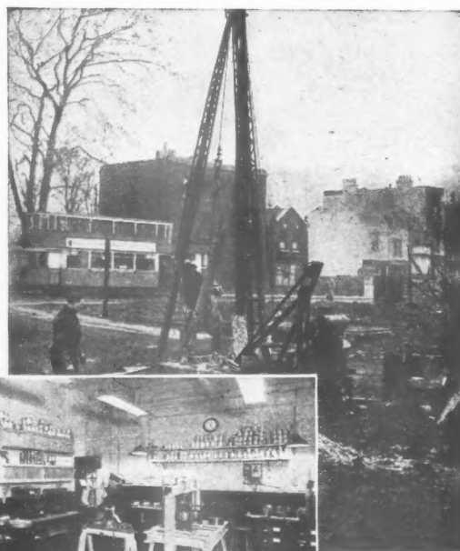
Test boring operations in progress.
