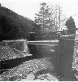
Left, a prestressed concrete bridge over the Heddon River Hunter's Inn, Lynton, Devon, designed by the County Engineers' Department. This bridge replaces one of ten washed out in the floods last year. The new bridge has a span of 40 ft. Construction is of hollow concrete trough units which have been placed end to end and prestressed by the Freyssinet system.
