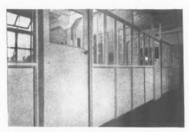
Offices constructed with 3-in. PLIMBERITE and timber framing, by Messrs. Batger & Co., Confectionery Manufacturers, London, E.I.
