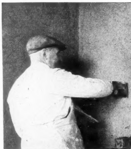
"ZONAPLAX" Undercoat Plaster being applied over brickwork in the usual manner.
