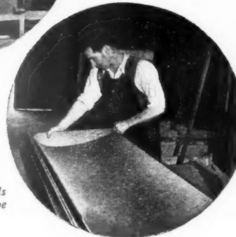
Sundeala boards can be bent to shape
