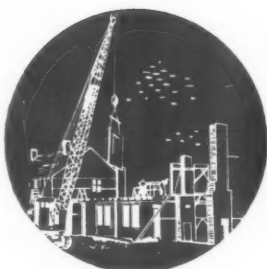
Illustration shows wall panel being hoisted in position.
