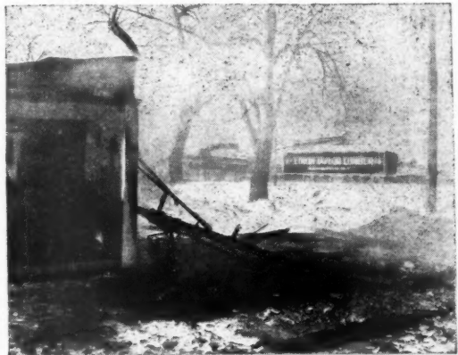
Same structure showing right hand side not treated with Albi-"R" completely burnt out and collapsed. Left hand side treated with Albi-"R" remains intact.
