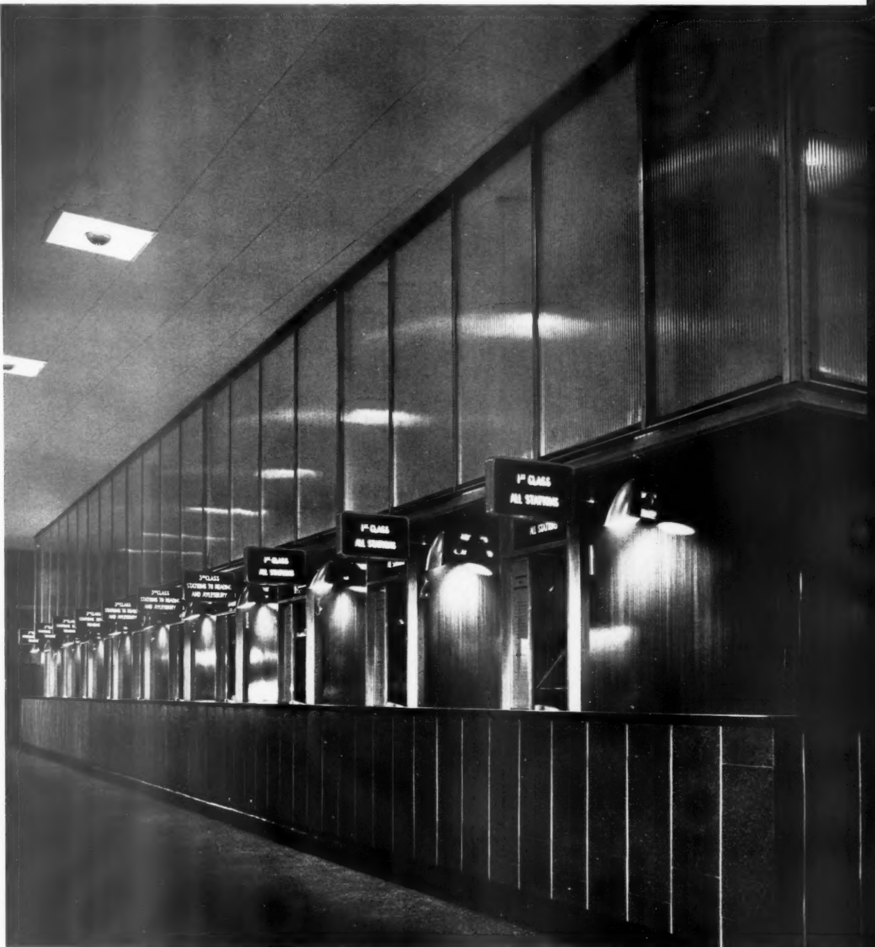
The panels between the ticket windows are of cellular plastic sheeting, veneered with sapele mahogany, and the large numerals are cast aluminium
