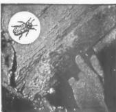
A rafter in the roof of Chichester of Chichester Cathedral showing damage by the Death Watch Beetle. Expert treatment of
