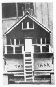
Somewhat less ridiculous is William Croxford's anti-flood house, seen above. It is floated on a pontoon and restrained by reinforced concrete piles.
