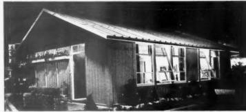
Left, a two-bedroom house, designed by J. A. Findlay of K.D. Homes (London), Ltd. The house on view is 776 sq. ft. in area and costs £1,265 f.o.b. The 4-ft. wide insulated panels are faced externally with steel on a timber or steel frame.
