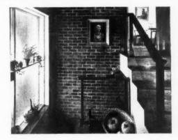
CONSTRUCTION and FINISHES.—External walls are of 11-in. load-bearing cavity brickwork, internal walls are of 4½-in. brick. The roof is covered with slates on battens and felt. Floors are of *in situ* concrete and precast concrete beams and hollow tile construction. Internally walls are plastered and finished with emulsion paint, with
