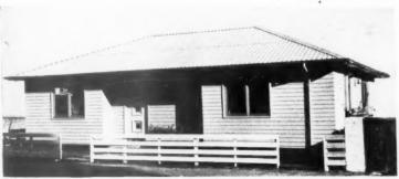
Left, the three-bedroom "Precut" house, designed by Frederick Cubitt and manufactured by R. Nerdrum, Ltd. The construction is of 2½-in. solid wood, with no framing, and the floor area is 920 sq. ft. This demonstration house is at Chelsea Square, S.W.3; the ex nibit at the BIF shows the system of construction.
