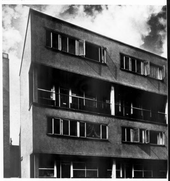
Reinforced concrete slabs, connected by columns, form the top and bottom of the balconies, the latter being a continuation of the floor which divides the upper flats from the lower
