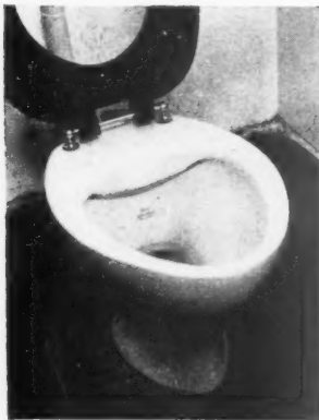
Figure 1. One of the latest developments in lavatory pans (Adamsez), showing, above, a clean-lined and attractive shape (which could be even further improved by corbelling), and left, the rimless bowl. The force of the flush can be adjusted at the inlet, so that the water cleanses the maximum area of the bowl without splashing over the edge. Thus any fouling is immediately detected, instead of forming under the rim, as in normal bowls.
