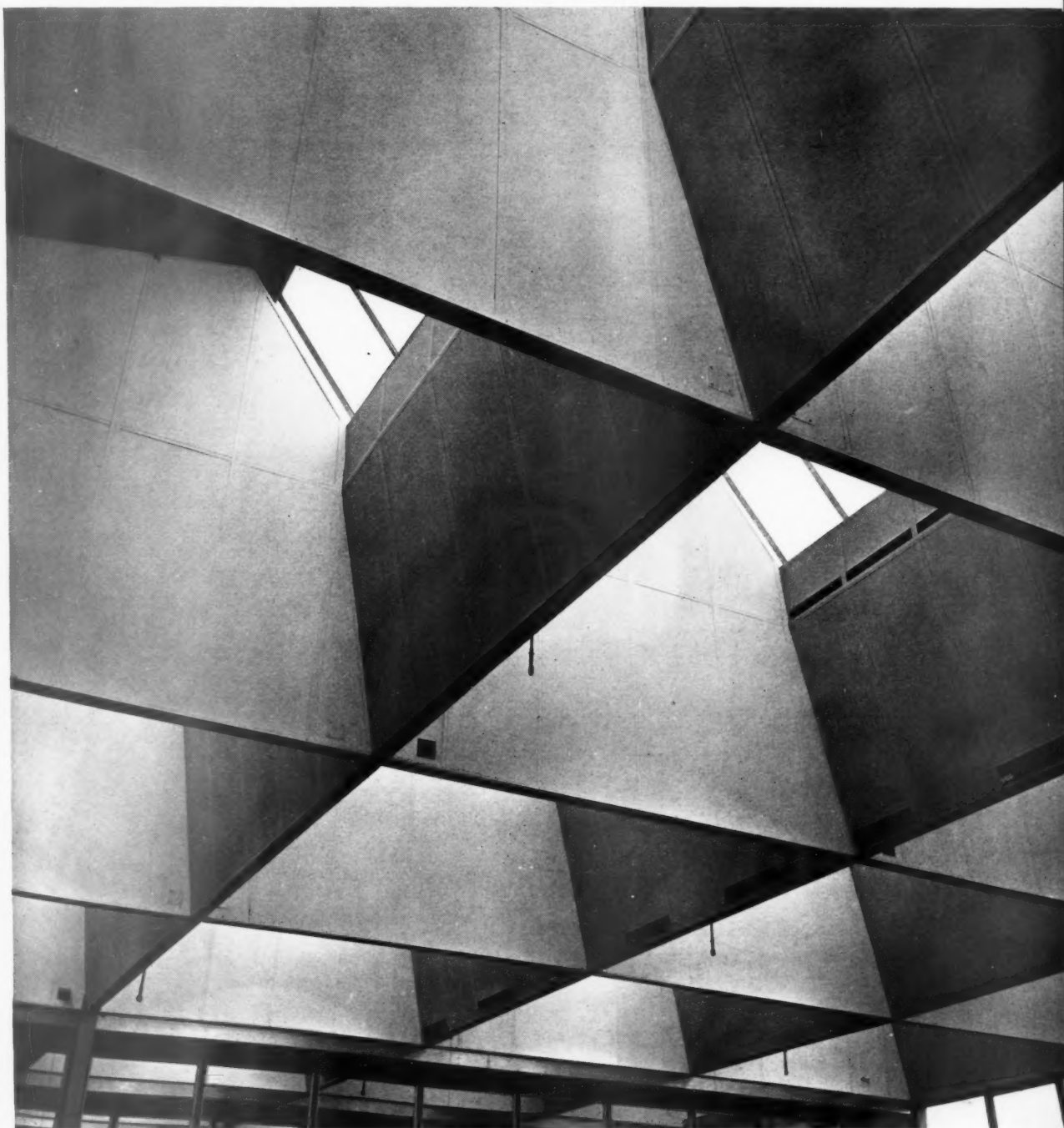
The fibreboard sheathing of the roof structural members, which diffuses the glare from the rooflights, also conceals the heating pipes
