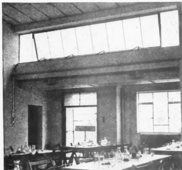
An H.H./M.H. Type 3 control fitted to a 16 ft. long top-hung window in the Canteen of the G.P.O. Stores at Brimsdown. Architect: Eric H. Firmin, A.R.I.B.A. Arens gear supplied by Aygee, Limited, of Perivale.
