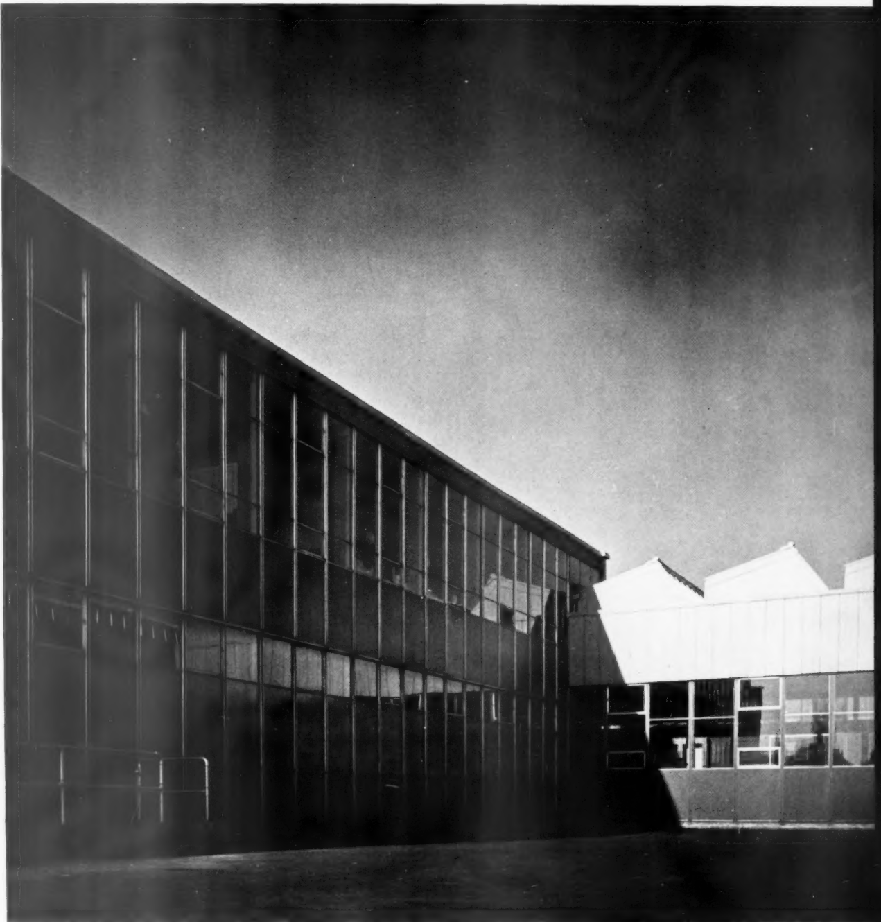
Pairs of light alloy connectors form the mullions which run the full height of the wall and support the plastic infilling panels and windows
