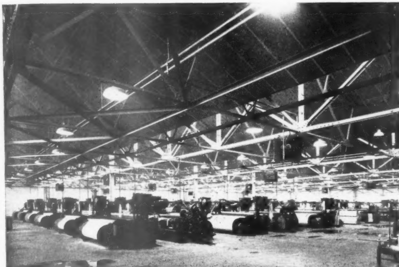
Fig. 7, traditional type roof trusses at the factory on the Aintree Trading Estate, Liverpool, designed by R. Bradbury, City Architect and Director of Housing.
