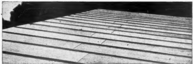
View of standing seam zinc roofing.
