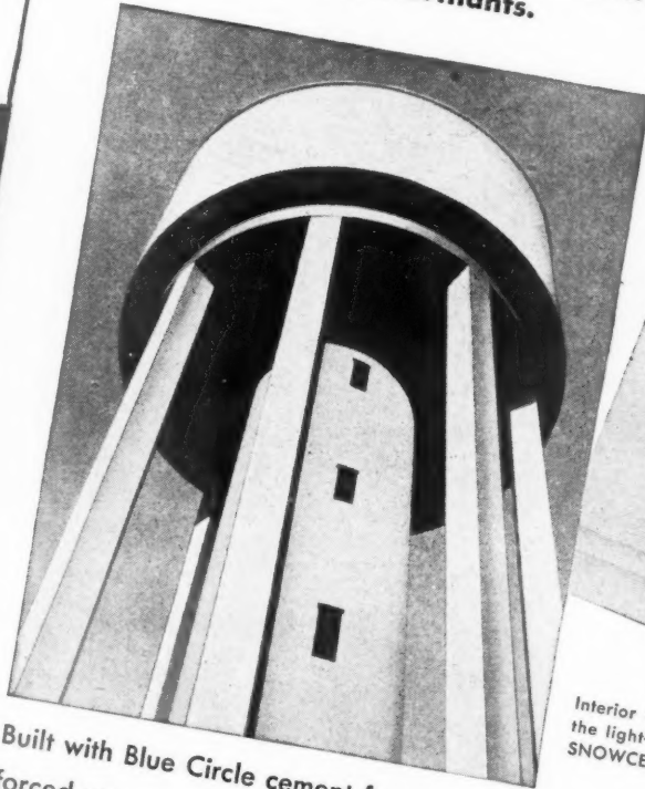
Willow Brook Water Tower, Corby, Northants.
