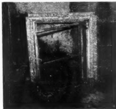
Standard hot-dip galvanized metal window undergoing corrosion test in the waters of Dover harbour.
