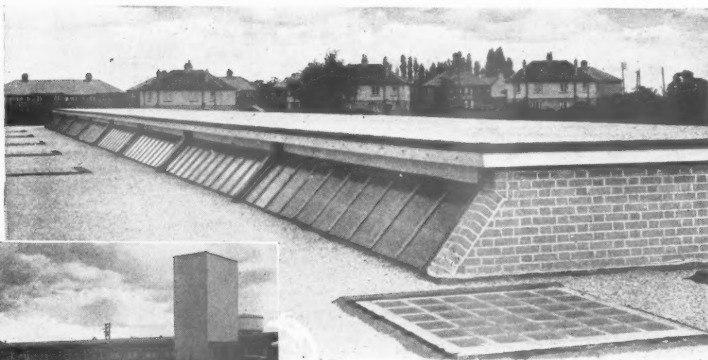
Hatfield-Dunville County Primary School for the West Riding of Yorkshire County Council. View of roof screeded with vermiculite.
