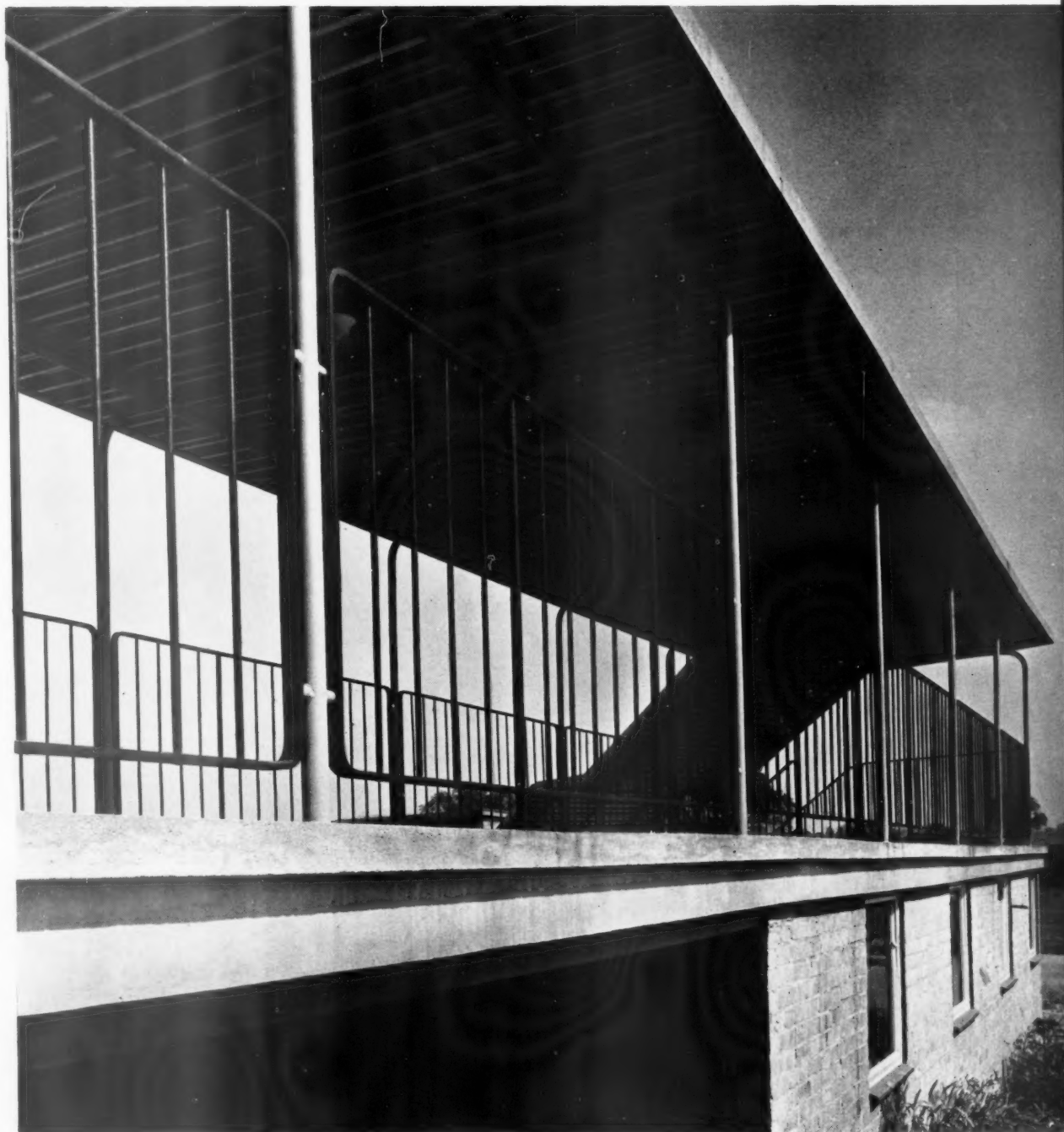
The roof to the covered way and staircase is of aluminium decking supported on tubular steel frames and purlins
