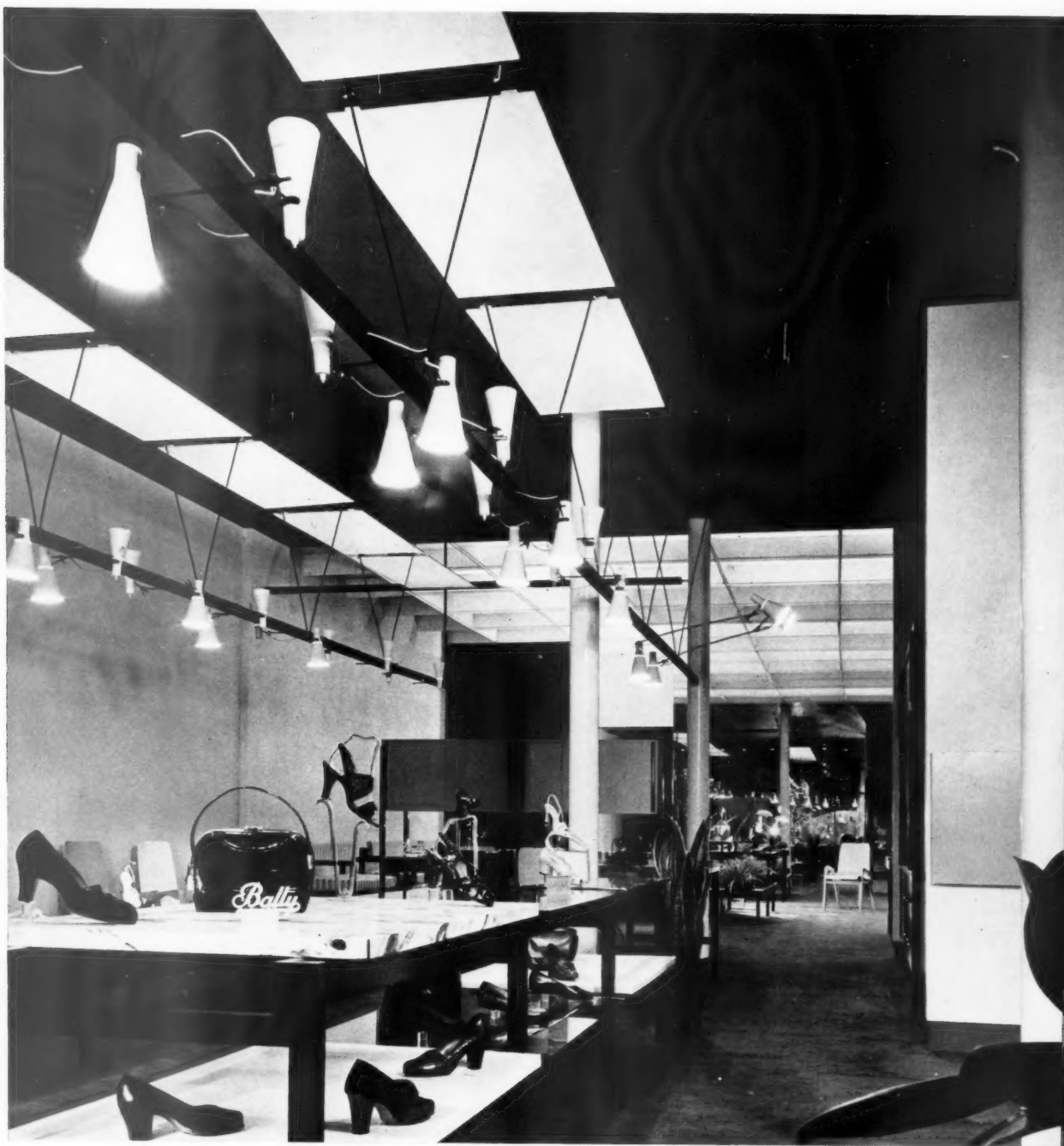
The radiant heating panels, which are painted yellow, and the adjustable light fittings are suspended by rods from the deep blue ceiling
