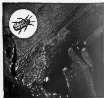
A raft in the roof of Chichester Cathedral showing damage by the Death Watch Beetle.
