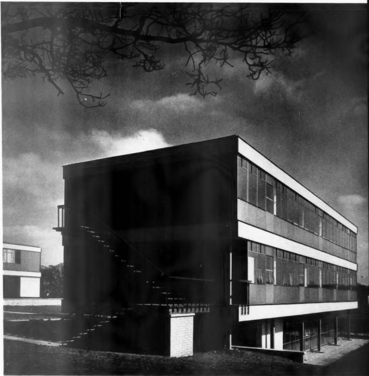
The walls, built clear of the stanchions, are composed of glass and cellular plastic sheeting in light alloy frames.
