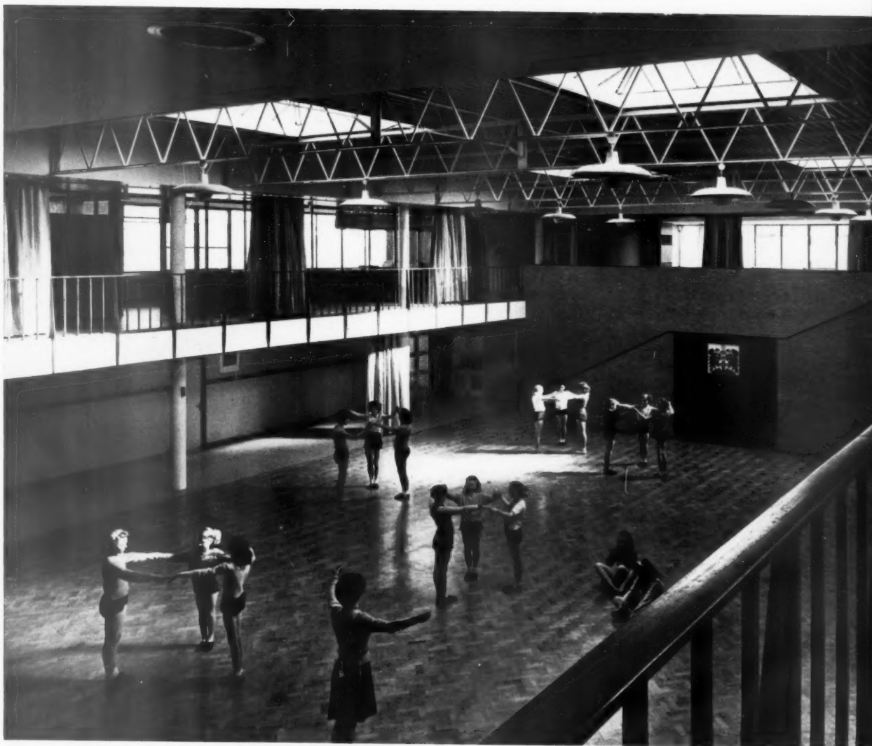
The shaped hardwood supports to the balustrade are notched over the edge of the balcony and are secured to the lattice beam behind the fascia.
