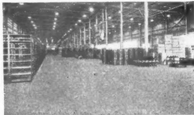
New Esso Refinery, Fawley. For Esso Petroleum Co. Ltd., Sealocrete Metallic Hardener used in concrete floors of the Central Maintenance Building. Contrs.: Messrs. Foster Wheeler Ltd.
