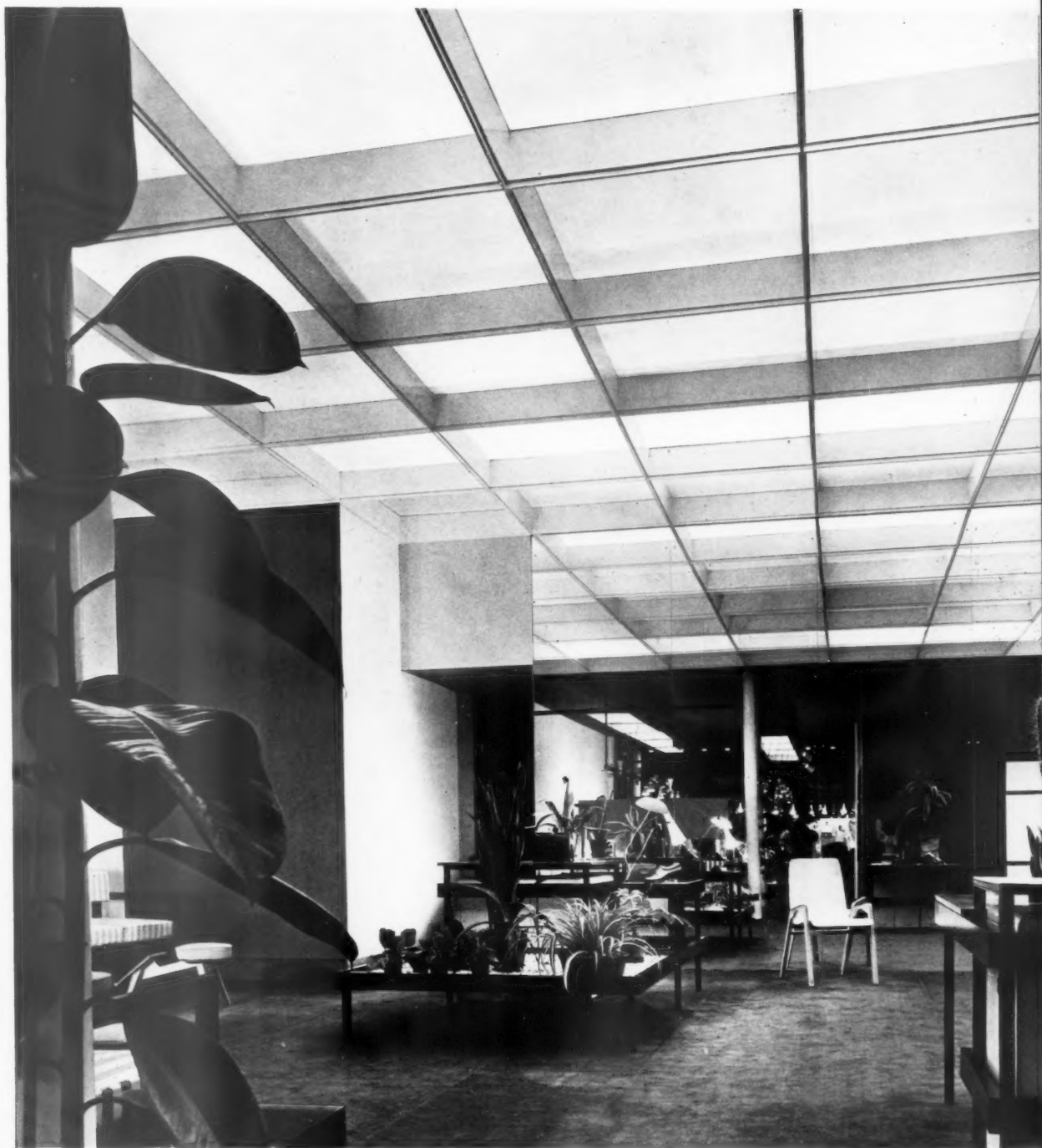
Three prefabricated panels form the laylight in which special diffusing glass is used.
