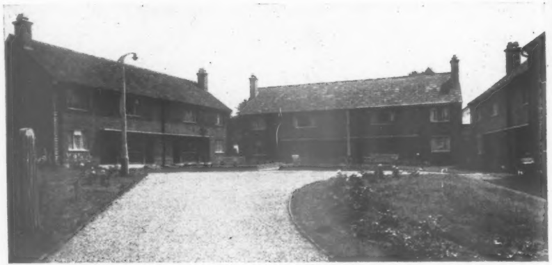
Flats at Finchley, London, N. 3
