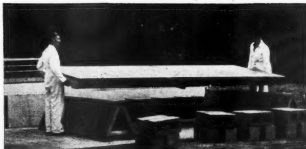
Above, section through standard "Trofdek" unit. Right, standard unit, 48 sq. ft. in. area, complete with "pre-fixed" flooring, being handled easily by two men. This unit, before being covered, was deflected only 1/10 of the span under the design load (30 lb./sq. ft.); it recovered, after loading for 24 hrs., 88 per cent. of the deflection; it failed at a total load of 14,500 lb (9½ lb./sq. ft.)
