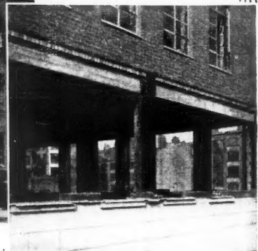
Illustration shows the use of Tretol Bitumen D.P.C. Membranes as used on vertical concrete columns, prior to "bricking in," and on concrete below ground level.
