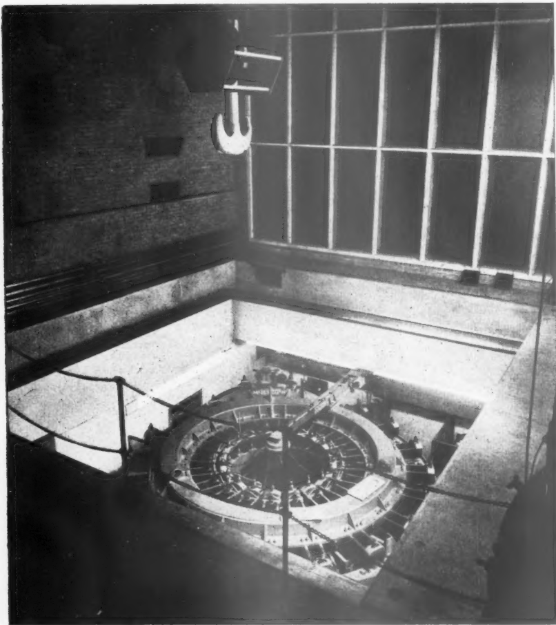
Left, the synchrotron hall, with the 150-ton sliding slab in open position. Above, the sliding slab closed over machinery when in operation. Below, control room, showing console for operating synchrotron and synchrotron hall window.
