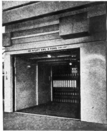
Vertically "bi-parting" (sliding) steel shutters: power operated: suitable for heavy-duty goods lifts.
