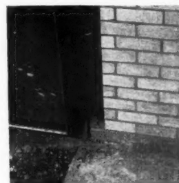
Close-up showing precise junction between brickwork and steelwork.
