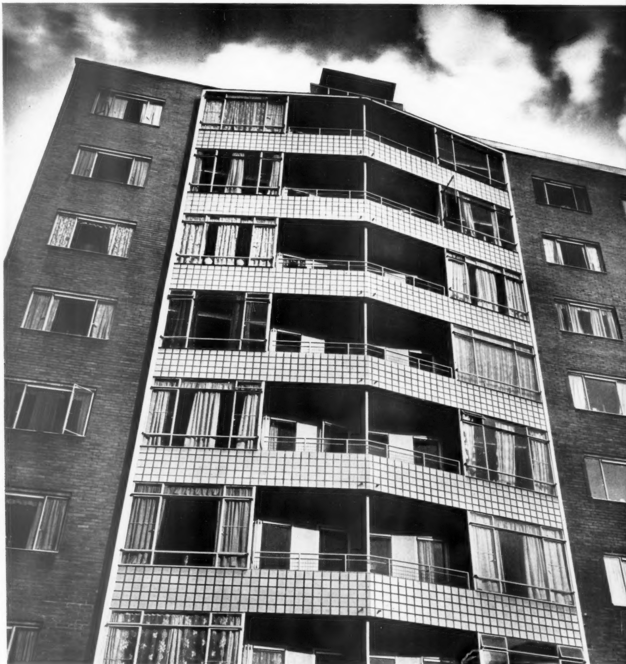
The facing to the balcony walls is of matt-glazed tiles with a waterproof pointing in the wide joints.
