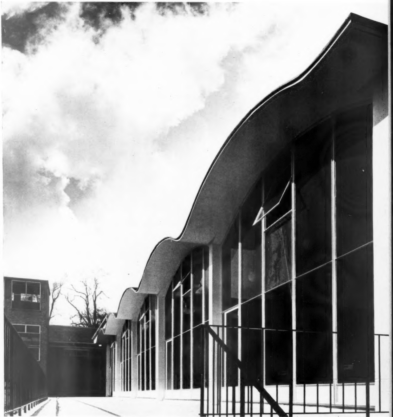
On the terrace side of the canteen the roof projects beyond an upstanding beam to form a wide overhang to the glazed wall.
