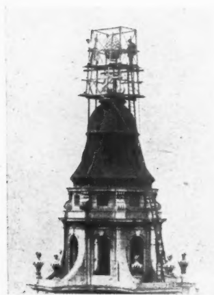
Fig. 8. A contrast. Traditional scaffolding on one of the west towers of St. Paul's compared with scaffolding in Premeditated Concrete.
