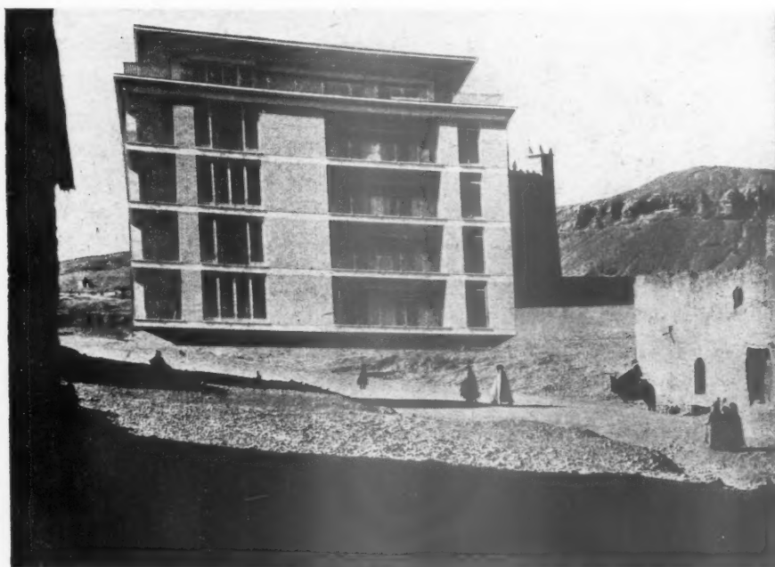
Fig. 6. A block of flats whose supporting columns or pilotis have been constructed in Premeditated Concrete.
