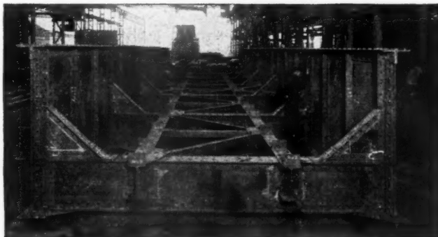
Single Track Railway Bridge in course of construction and trial erection prior to shipment overseas.
