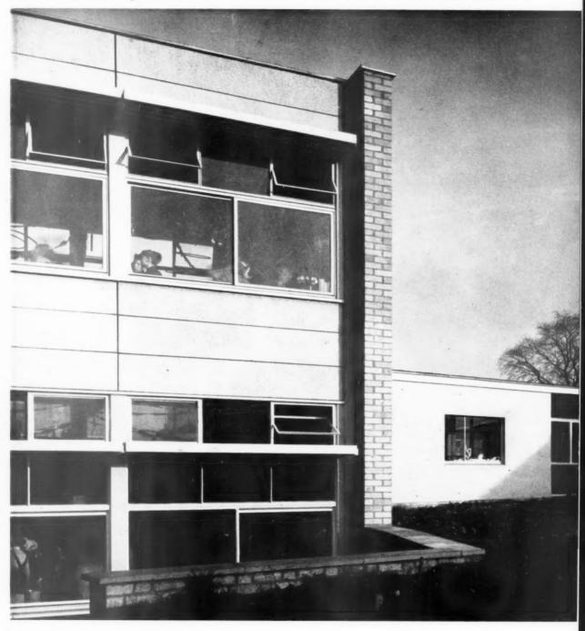
The chief interest in this detail centres around the hard-wood sun-baffle and in the flashing which was required at the point of junction of its supporting bracket with the stanchion. The precast concrete slabs which comprise the cludding are attached direct to the stanchions at points which do not appear on the drawings.
