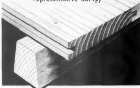
We recommend the P.T.G. boarded filleton-concrete floor, pressure treated with 'TANALITH' preservative as having the following advantages.
