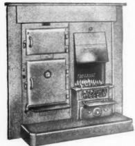
The "XL-TALBOT" is an entirely new design of the popular 38" × 38" Side-oven Combination Grate, being continuous burning on Coke, Coal or any other solid fuel. It gives an open or closed fire as desired, providing an abundant supply of hot water, with ample cooking facilities.
