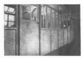
Offices constructed with 3-in. PLIMBERITE and timber framing, by Messrs. Batger & Co., Confectionery Manufacturers, London, E.1.
