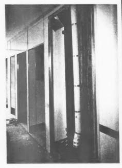
Left, central corridor in south block. Above, typical vertical duct with laminated plastic panel removed to show services. Bottom right, typical examination cubicle.
