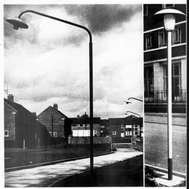
In the standard on the left, the bulb is protected by a casing of expanded aluminium lathing. The standard on the right, which is more formal in character, is fitted with a glass globe. In this example the junction box is positioned directly above the light.
