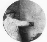
GYPLITE Undercoat Plaster being applied over brickwork in the usual manner.
