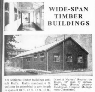
For sectional timber buildings consult Hall's. Hall's standard 6 ft. unit can be assembled to any length in spans of 10 ft., 12 ft., 15 ft., 18 ft., 24 ft. and 30 ft. Built throughout of selected, fully seasoned timber (Hall's have their own timber drying kilns) they are widely used as Classrooms, Village Halls, Community Centres, Recreation Rooms, Canteens, Factory extensions, etc. Fully detailed plans supplied against your specification.
