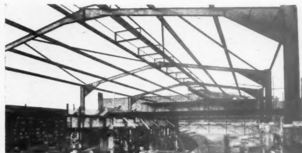
Transport Depot with Two Ton Crane at Midspan.
