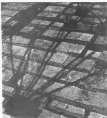
Ductube forming ducts in hollow pot floors, for complete lighting and power layout, terminating in consumer panel.
