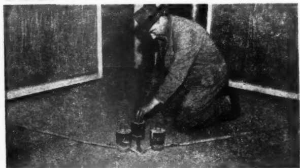
Part of wiring circuit with Ductube laid over MYKO floor before final floor topping.
