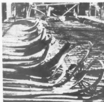
Formation of electric installation ducts. Note simple method of bending even larger sizes. Laying took only 1½ working days against estimated time of 1½ weeks for metal conduit.
