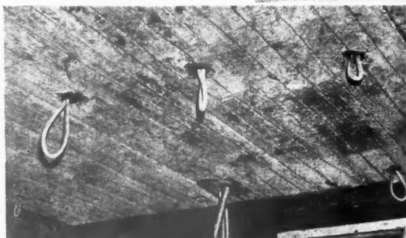
Underside view of precast concrete floor beams showing Ductube looped through B.S.S. ceiling point fittings.
