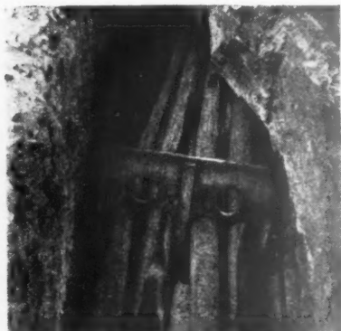
Left:— 4 Ductube forming 6 way electric cable ducts at a Power Station in Algeria.
