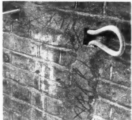
Example of Ductube forming duct in chases let in a brick partition wall to supply B.S.S. wall fittings.
