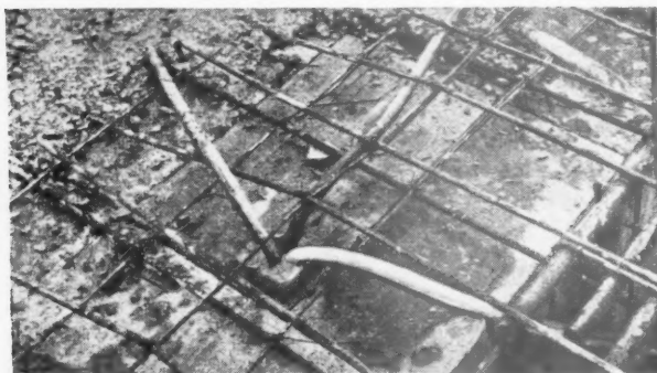
Ductube used to form ducts in 5" "in situ" concrete floors.
