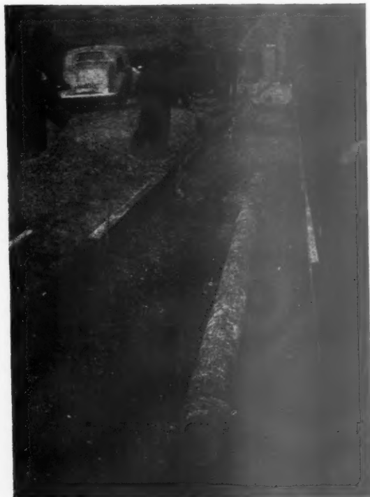
9 Ductube forming surface water drains in Hampshire
