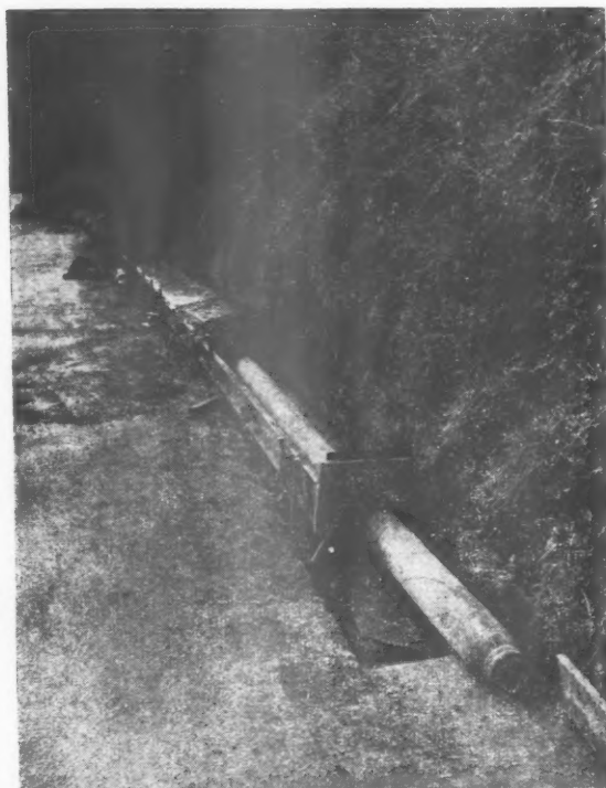
Right:— Ductube used for surface water drains in Dorset.
