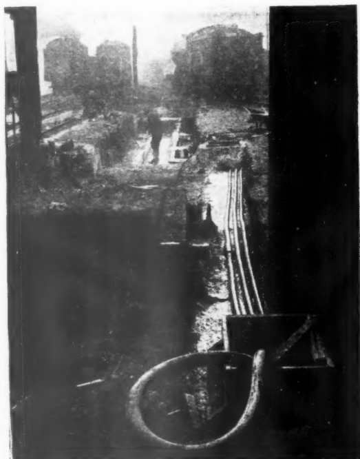
3 DIA Ductube used in the reconstruction of Engine Pits at Stratford, to form 3" ducts for pit lighting cables.
