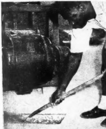
Ductube used with plastic conduit for turning up to socket outlet position.
