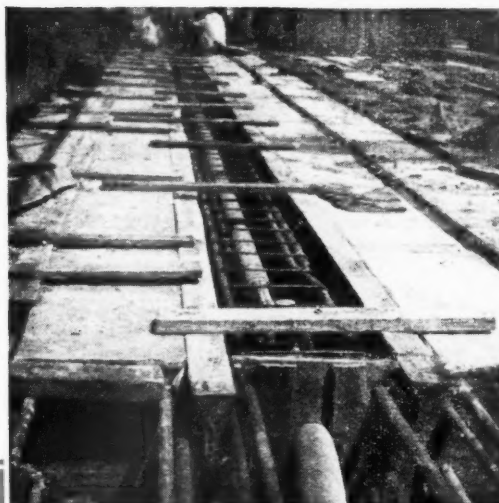
6 DIA Ductube being used for the construction of 80 ft hollow piles in Bombay.
