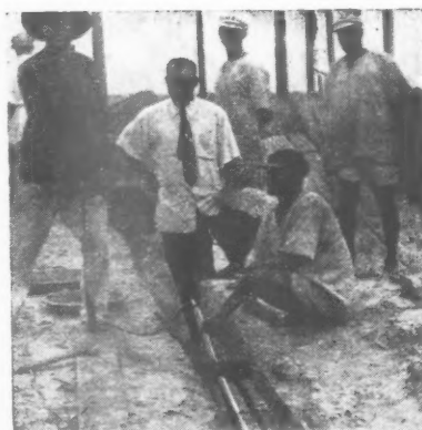
Right:— 4 Ductube in use for cable channels at a Power Station in Nigeria.
