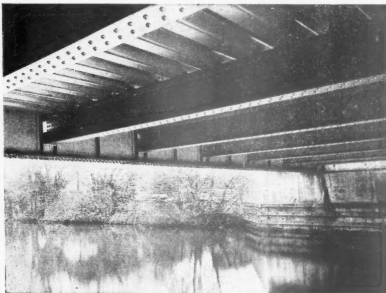
Bridge at Southall over the Grand Union Canal, jenolized and painted by Struc-Steel Painters Ltd., Isleworth, for the Borough Engineers' Department, Southall.
