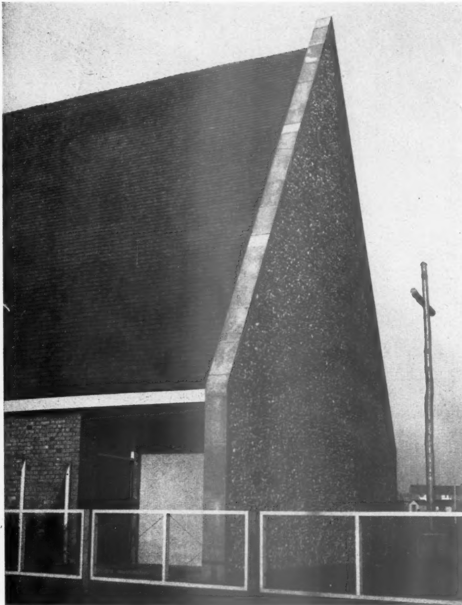
Left, the east wall of the chapel, which is flint faced. On the right is the rough fir cross, constructed from a tree which had to be removed on a nearby development. Below, a general view of the hall looking towards the chapel.
