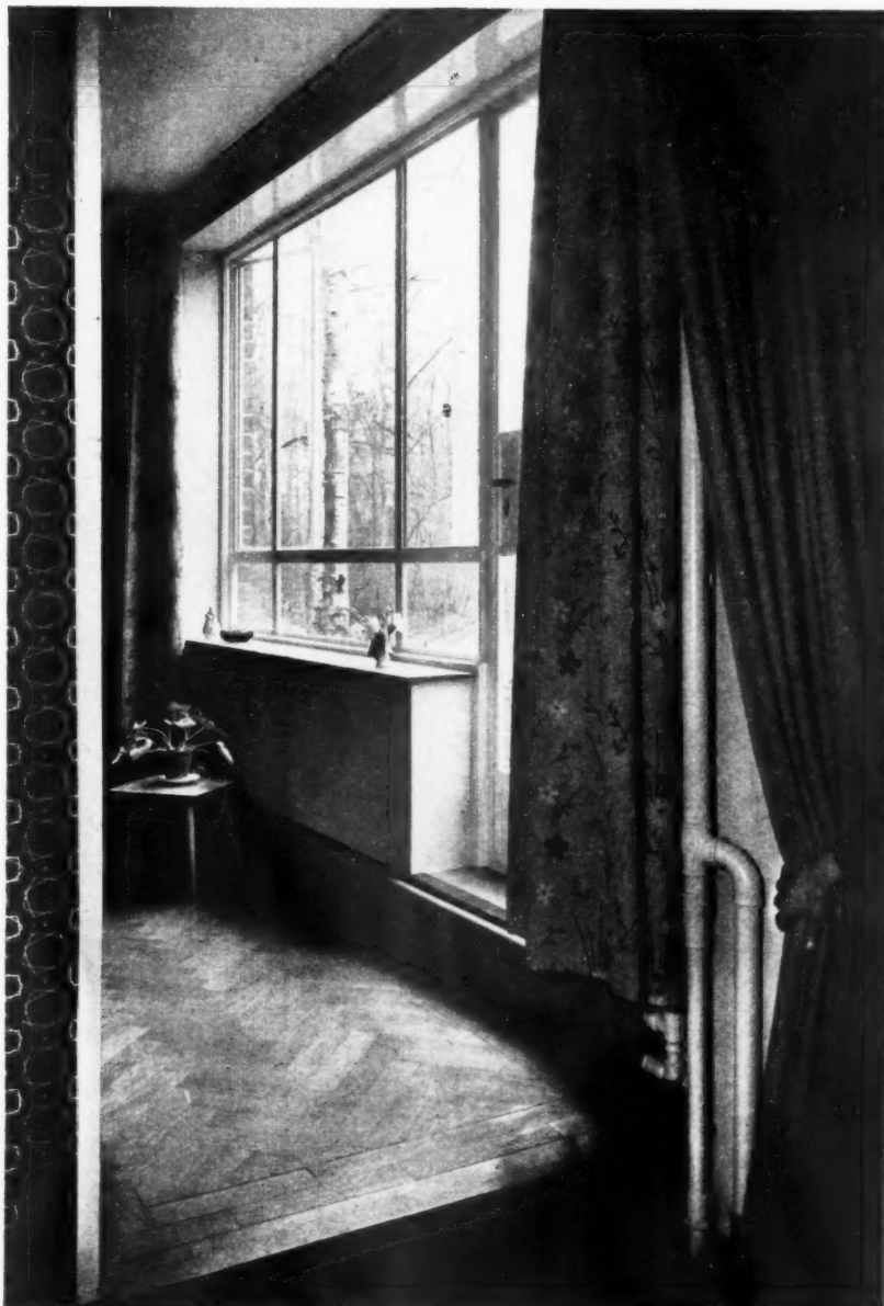
Fig. 4 (above). Main return pipe serving the dining room and living room circuits. Fig. 5 (below left). Cover plate on angle. Fig. 6 (below right). Valve for controlling radiator.
