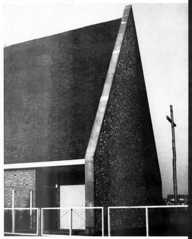
The flints have an average width of 2 in. to 3 in. and length of 4 in. to 6 in. and were laid in courses as the brickwork proceeded. The internal face of the brick wall is English bond, the external face header bond. The use of the large number of bats required by the splay and the batter served to give a more efficient key to the mortar.
