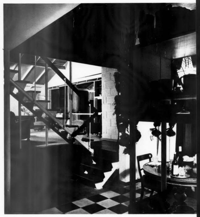
The tubular strings, the straps to support the treads and the standards supporting the handrail were shop-welded and the measuring for the handrail was carried out after the stair was fixed in position. The spacers on the opposite side of the main flight from the handrail are bolted to the rolled steel sections and the upper ends of the main strings are secured by coachbolts to the underside of a filler joist.
