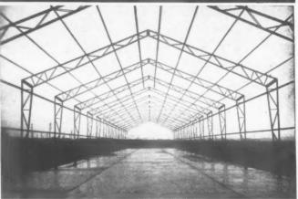
Standard Steel Framed Building Height to Eaves. 8ft., 10ft., 12ft... IOft., 12ft., 40ft. oft ... 50ft. 8ft., 10ft., 12ft., 60ft. 8ft., lOft., 12ft., 15ft. Lean-to and Canopy extensions are also supplied at standard roof slope of I in  $2\frac{1}{2}$ .
