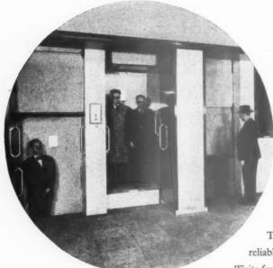
The recent installation illustrated consists of three Paternosters serving seven floors. Each car holds two persons comfortably and is capable of transporting 600 persons per hour in each direction.
