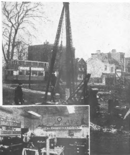
Test boring operations in progress.
