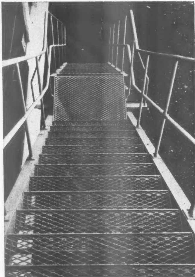
"Expamet" Openwork Stair Treads at London Airport Engineers: Messrs. Allen & Greaves, Ltd. Contractors: Messrs. Holland and Hannen & Cubitts, Ltd.
