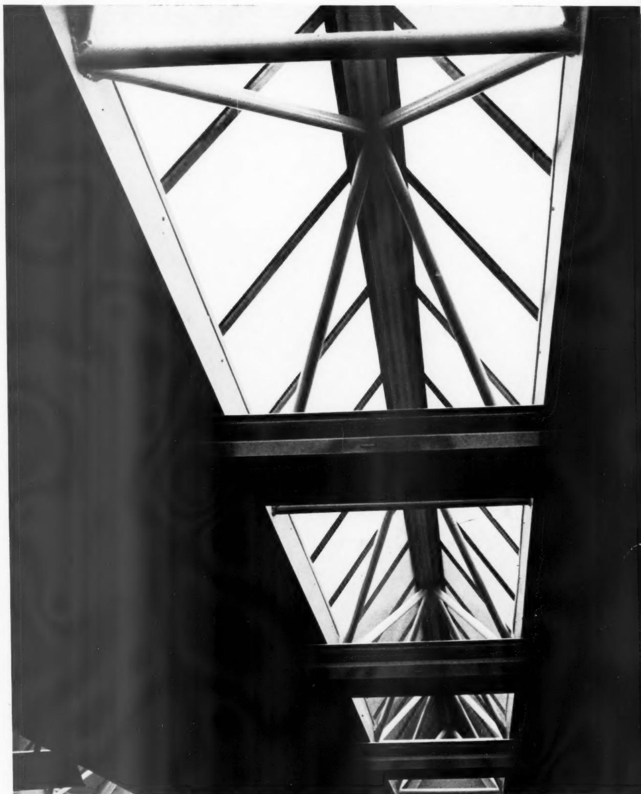
The tubular space frame spans 40 ft. and supports both the rooflight and the adjoining decking. Steel angle purlins are welded on either side of the apex of the frame to hold the standard patent glazing.
