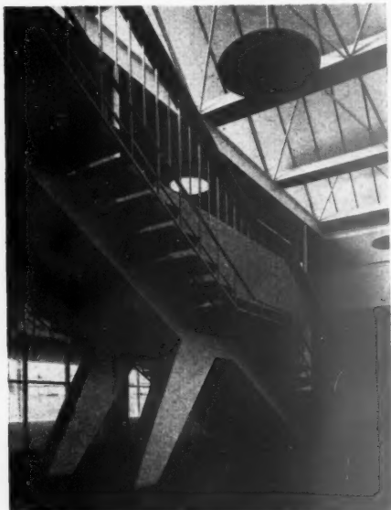
Above and above right, staircase on the west side of the crush hall, which is lit by aluminium framed patent glazing carried on tubular steel space frames. The double-swing sliding doors between crush and assembly halls will be illustrated later as a Working Detail. Right, the craft room, which is the only teaching space on the ground floor of the main block. Bottom, cycle store on the south side of the school.
