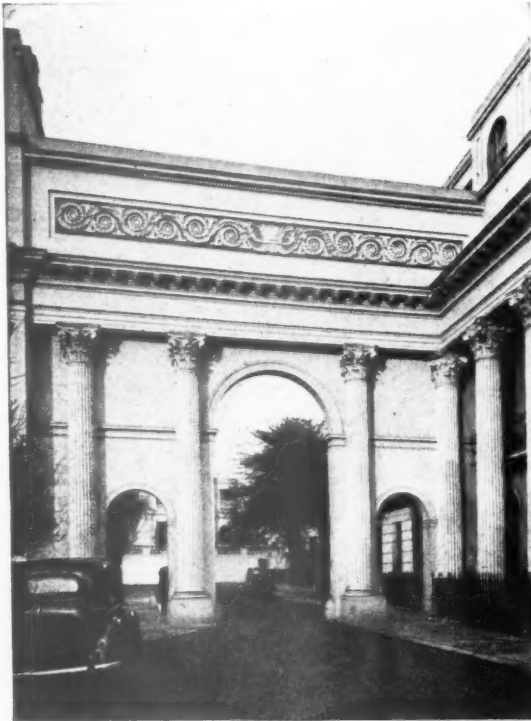
Friezes at either end of Chester Terrace Archways
