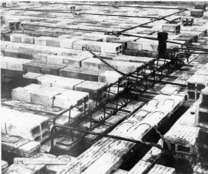
Left: upper floor of lavatory bay (11 ft. 3 in. span), of in situ concrete to facilitate placing of soil connections.
