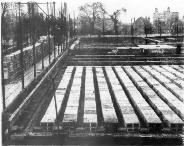
Left: upper floor adjoining stair-well. In the background: centering ready for plank laying. Note blocks fixed to shutter at edge of floor to form holes for bronze cramps for the slate facing. Note also electric conduit built into 9-in. wall.
