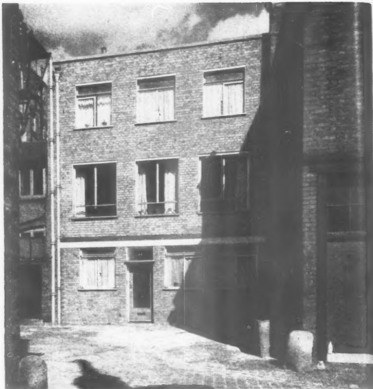
Above, the rebuilt west facade. The beam over ground floor windows spans the original opening for a double garage.
