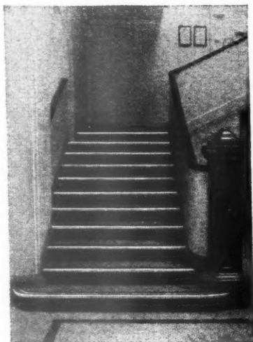
PHOTOGRAPH DON Plastic-filled Stairtreads in use on the staircase of a Government Department in Bristol. The ribbed surface of the plastic
