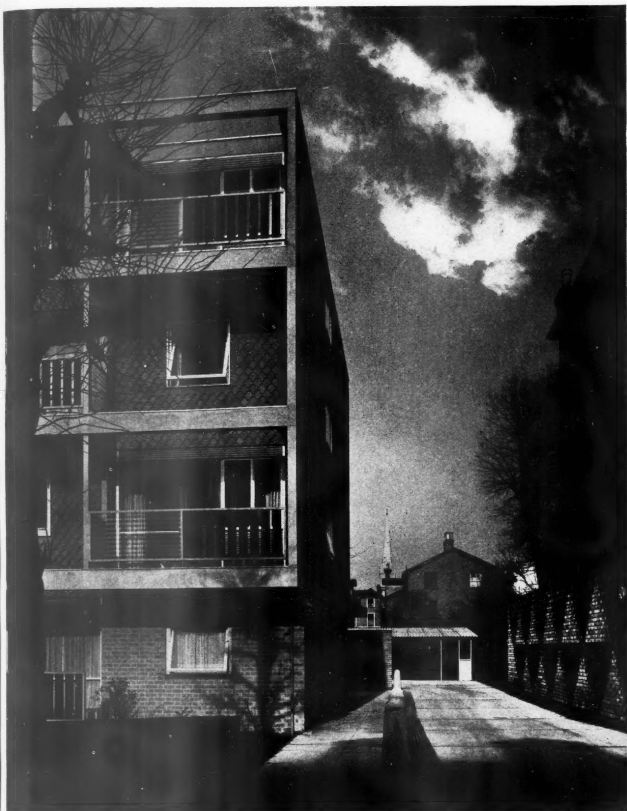
Detail of the street elevation. Construction is generally of load-bearing brick but concrete floor slabs are cantilevered as staggered balcony floors and are joined by horizontal concrete ties. The vertical end members are rendered clay conduit blocks with steel reinforcement.
