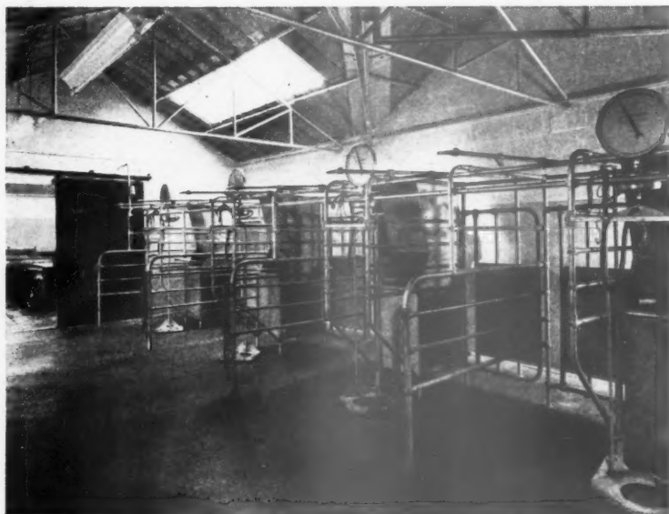
Top, from the south. On the right is the milking parlour and dairy. Above, the milking parlour looking towards the dairy. Below right, the dairy. The floor is granolithic and the asbestos cement roofing is carried on tubular steel trusses.
