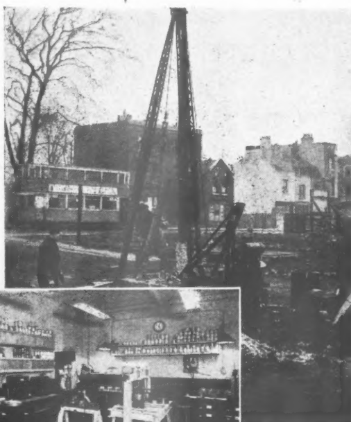
Test boring operations in progress.
