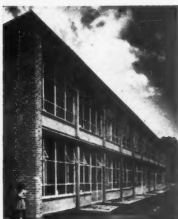
Top, the assembly hall, which has a roof carried on light welded steel trusses. Above, south facade of the two-storey classroom wing. Panels under windows are of common brickwork, rendered and painted blue. Facing bricks are sand-faced, straw coloured.
